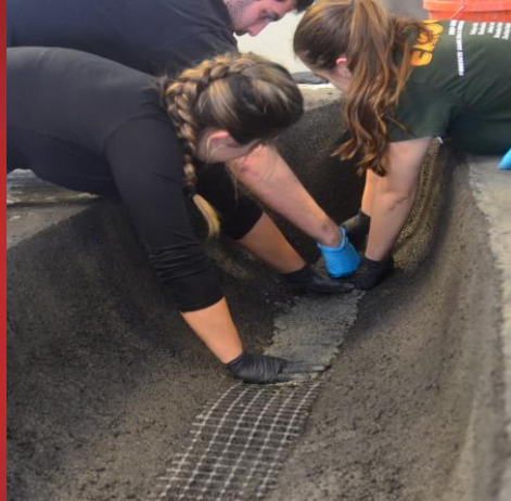
Figure 42: Reinforcement spine & structural layer.
