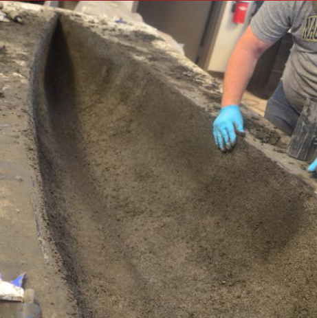
Figure 41: 1st finishing layer.
