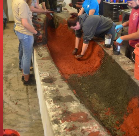
Figure 43: Final reinforcement & 2nd finishing layer.
